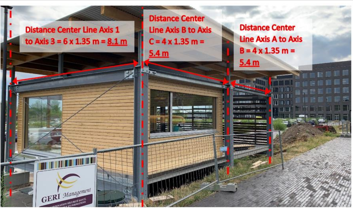
Figure 8: Indication of maxi grid axis of the columns, only the grids in axis A, B and C of Figure 7 are shown.
